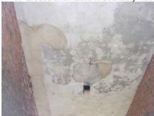
5. Eroded brick faces to boundary wall
