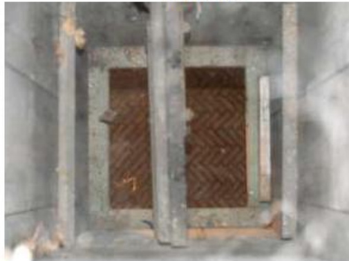
26. External polycarbonate sheet and window mullions damaged by vandalism.
