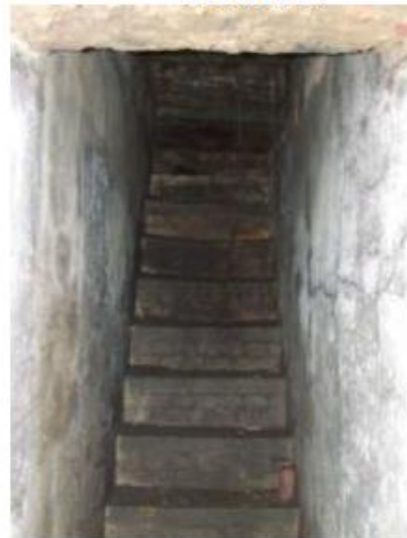
42. Additional access stair, now sealed, comprising brick risers with stone treads.
