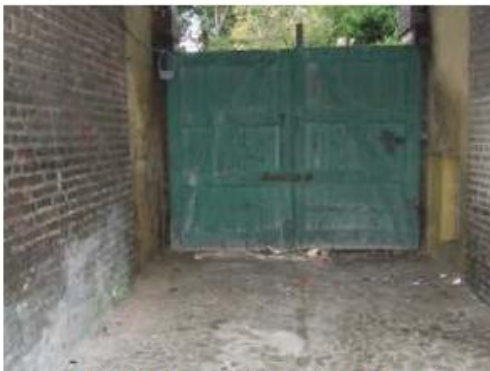
31. Timber double gate adjacent western stable
