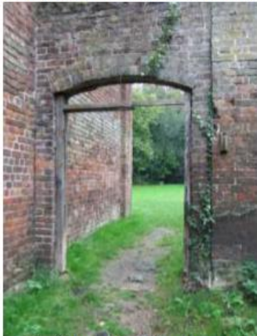
3. Adjacent wall and opening
