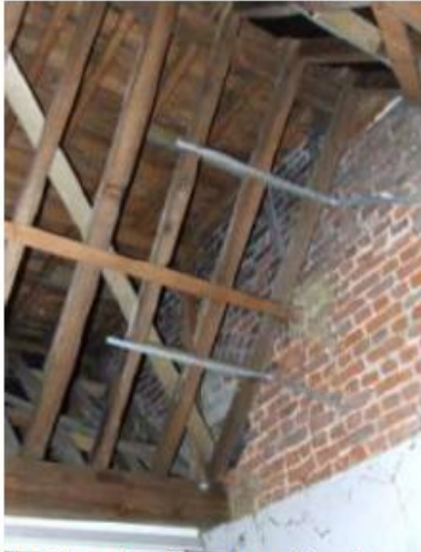
25. Galvanised straps utilised to secure roof timbers
