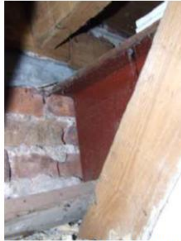
30. New steel RSJ bearing on internal blockwork skin.
