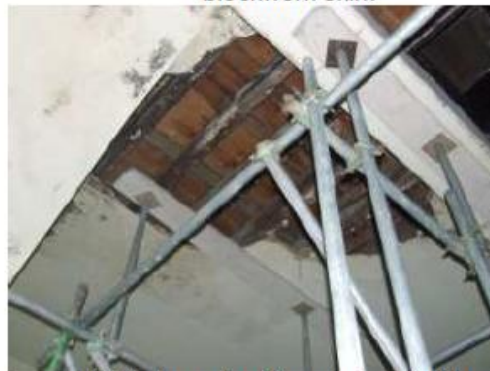
32. Collapsed ceiling and scaffold support in western stable
