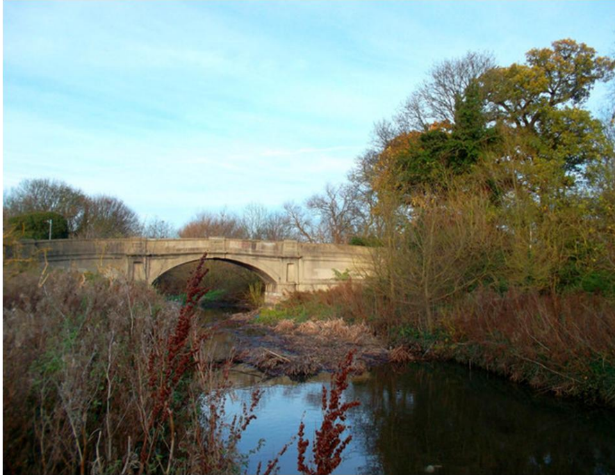
View of the driveway bridge from the south, by A. Lad 2014
